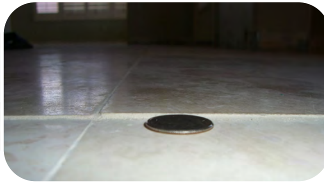
LIPPAGE (UNEVEN TILES)
